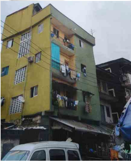
The five storey building at No. 63 Massey Street, Ita Faaji, Lagos Island before it went down
