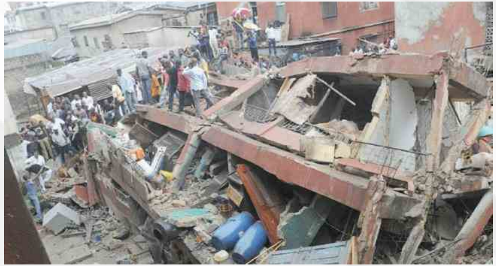
When the building collapsed
