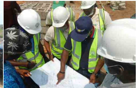
Visit to Ministry of Housing 300 unit residential project site at Kobape.
